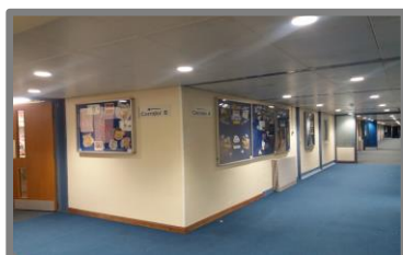
Shaftesbury High School – new LEDs
